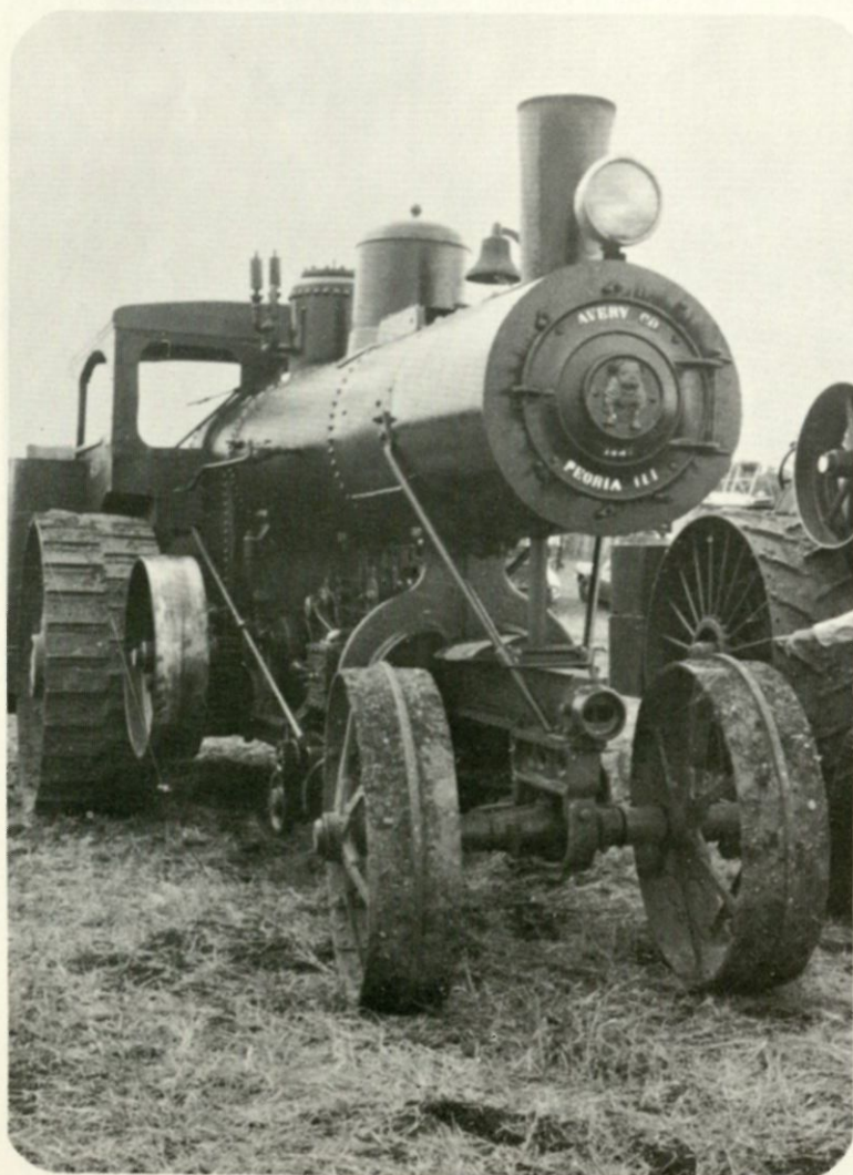
22 h.p. Avery double cylinder undermounted plow engine. The only engine on the grounds with 2 speeds forward. This heavy traction engine was built in 1912.
