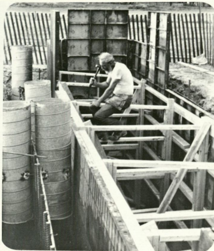
Forming the wheel pit on a hot 4th of July.
