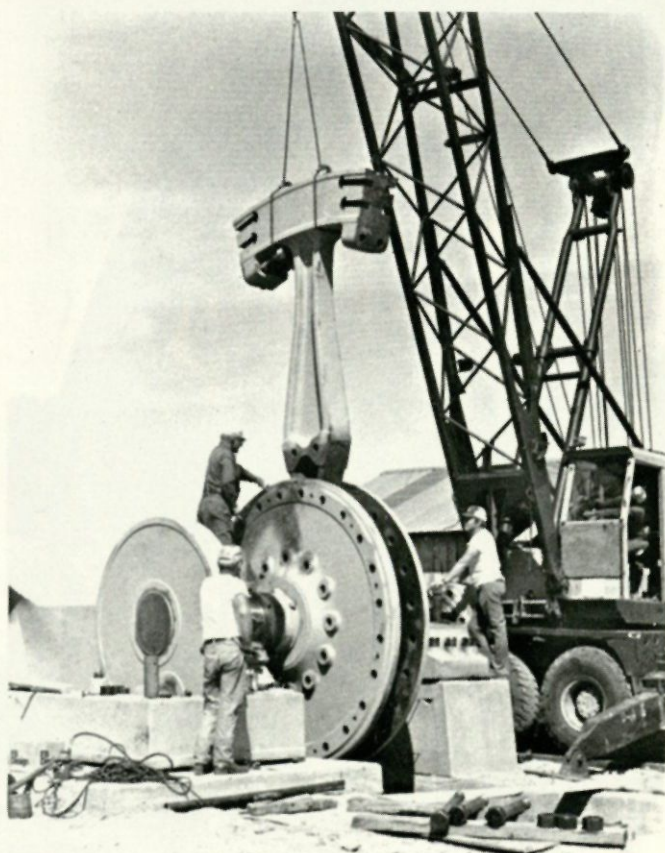
Aligning No. 1 spoke.
