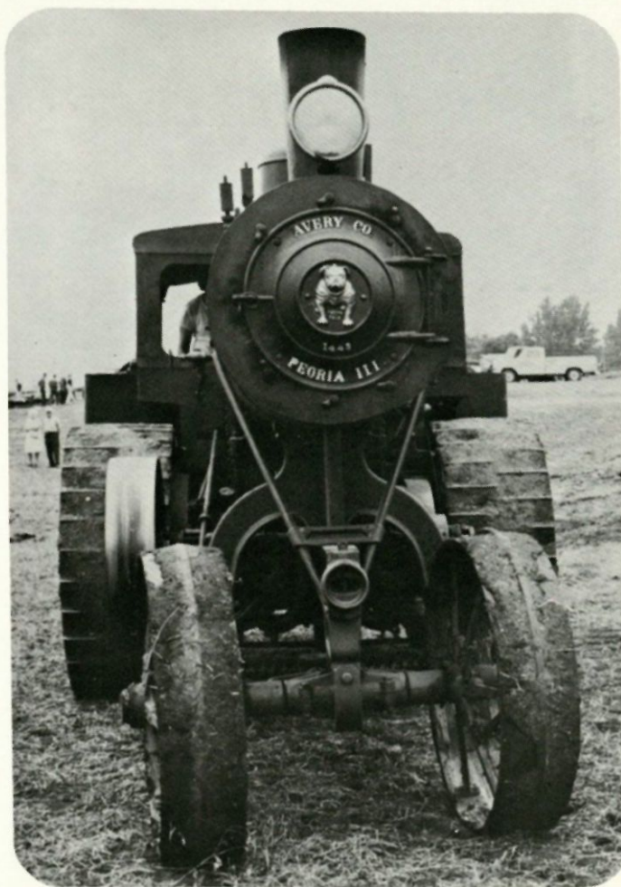
Henry Johnson's 22 h.p. undermounted Avery plow engine.
