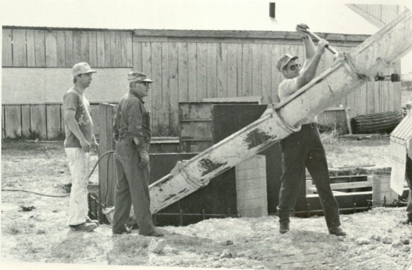
Pouring the first of 100 plus yards of concrete.
