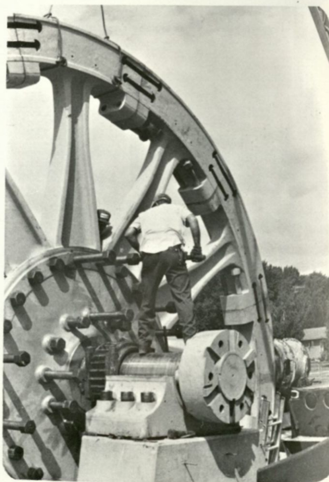
Driving in the 80 lb. bolts which hold the spokes in place.
