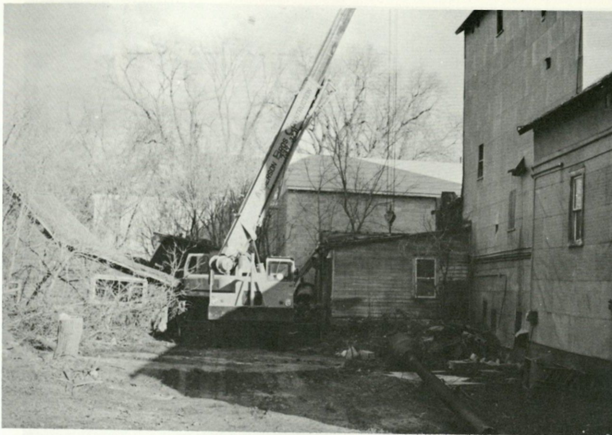
Getting ready to pull cylinder out through the roof.
