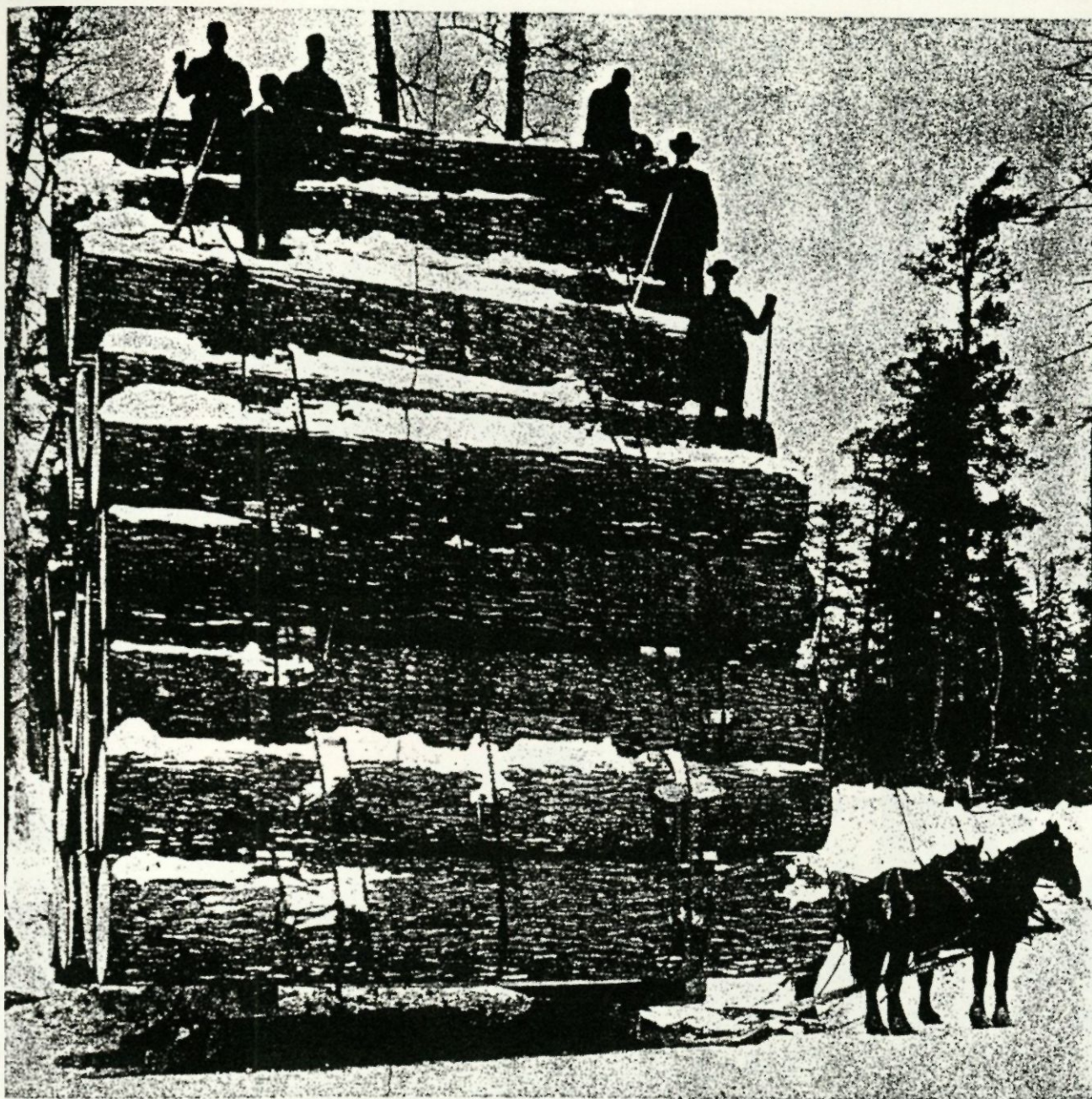
This load of logs on 16 ft. long sleigh bunks was hauled February 26, 1893 to an exhibit at the World's Fair in Chicago. It consisted of 144 tons of 18 ft. long white pine, scaling 36,055 ft., and was the largest load of logs ever hauled by one team. The haul to the river was three miles, over an ice road. The height of the load was 33 ft. 3 in. Nine flat cars were required to convey the logs to Chicago.
