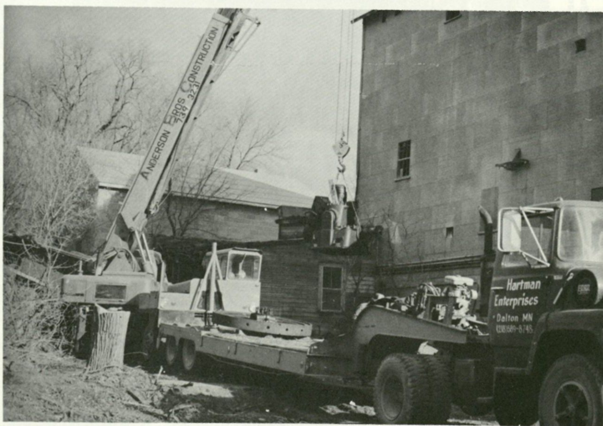
Loading the base of the 75 h.p. Fairbanks Morse onto the trailer.
