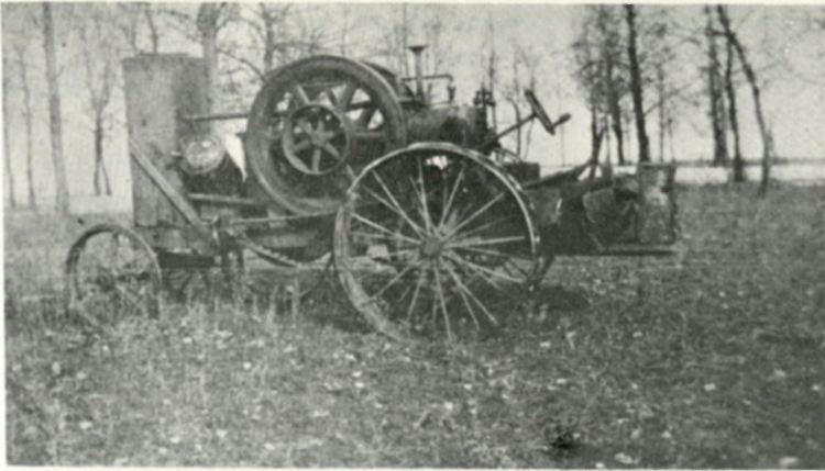
Home built tractor made by George Melby around 1920. The drive wheels are from a binder and the engine is about a 6 H.P.
