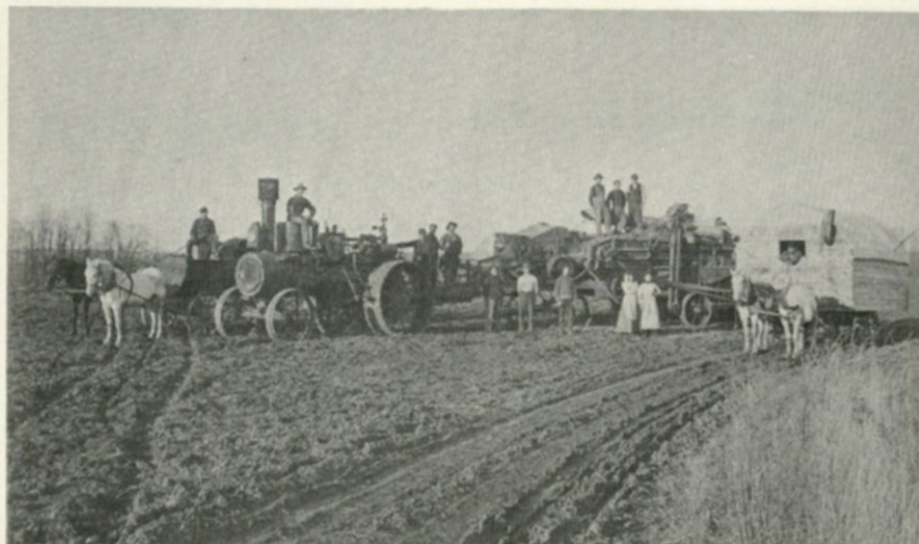
Picture of Nicols & Shepard steam engine and grain separator taken sometime around 1910 near Kensington, Minn. Note the cook shack and cooks. They fired with straw in those days as it was cheap fuel. The farmers had plenty of straw and there were no questions asked. Note the screen on top of the smokestack. That was used to catch the sparks so they would not set the stack on fire.
