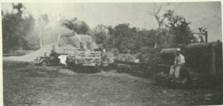
Threshing in 1940. 65 h.p. Caterpillar tractor and 36 x 58 Minneapolis separator. Picture was taken at the Dick Waltjers' farm on the north shore of Ten Mile Lake. R. J. Melby is the present owner of the rig.
