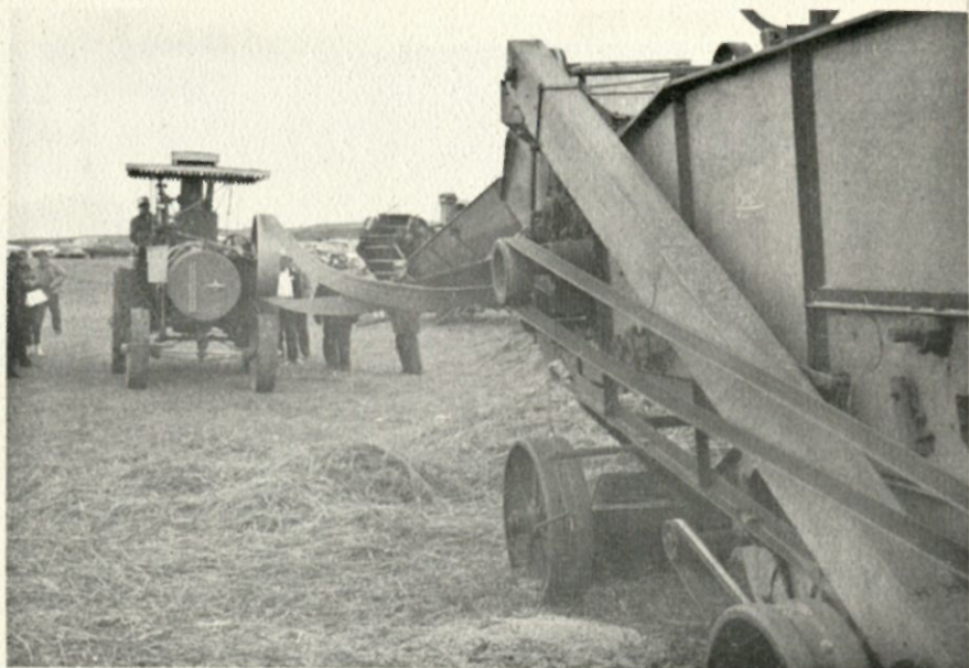
24 h.p. Kitten steam engine belted to a Case separator at Dalton's show.
