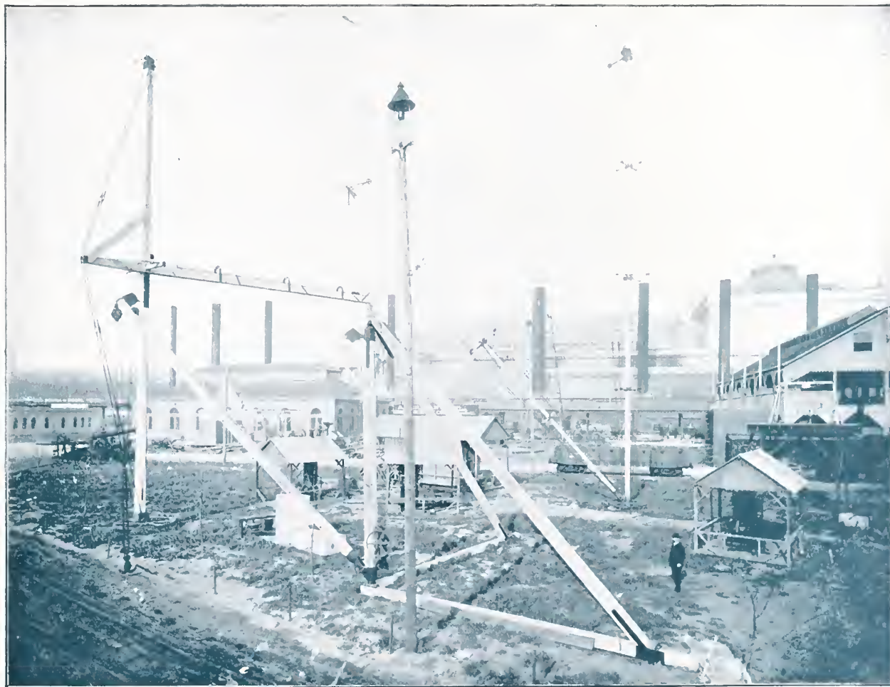
Cut 343. AMERICAN HOIST & DERRICK CO.'S EXHIBIT, WORLD'S FAIR—THIS EXHIBIT TOOK THE MEDAL. Tubular Guy Derrick—Mast, 80 ft. Boom, 75 ft. Capacity, 10 tons. Crane Derrick—Mast, 65 ft. Boom, 50 ft. Capacity, 5 tons. Stiff-Leg Derrick—Mast, 30 ft. Boom, 40 ft. Capacity, 8 tons.
