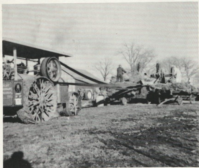
Avery steam engine and separator threshing in 1959. Avery built straight flue, return flue and undermounted steam engine and also the Avery yellow fellow grain separator.
