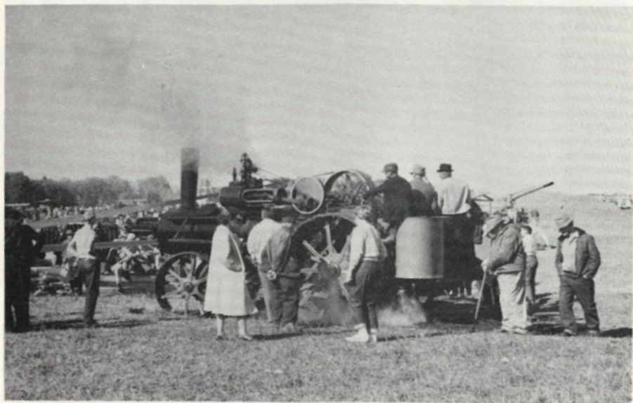
25 H.P. Wood Bros. steam engine belted to the saw mill. Very few Wood Bros. engines are left in the country. The company didn't make many engines. They started late in the game of building steam engines. They built a 30 H.P. double gear engine. We don't know if any of these engines are left.
