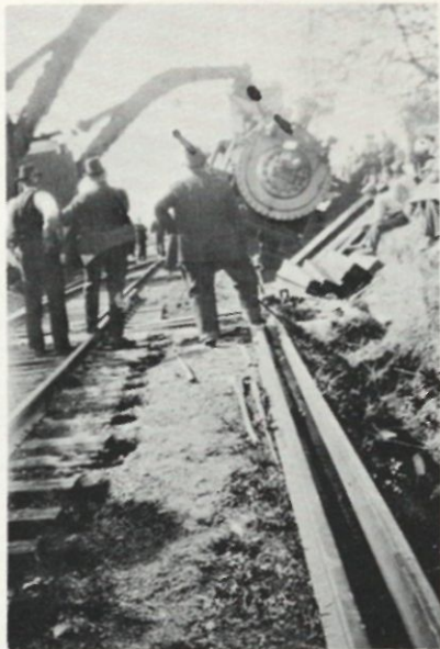
Locomotive engine that jumped the track and tipped over on its side at the side track in Dalton. The train was switching in gravel cars for paving Highway No. 59, but too much gravel and rocks got on the track and forced it off the rails. Year, 1937.
