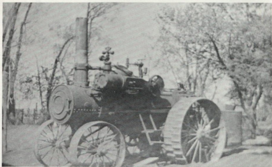
16 H.P. Advance steam engine, new about 1905, was owned by the late Wm. Pennie, Villard, Minn. Was used for threshing, lumber sawing, silo filling and feed grinding. It was replaced in 1925 by a 20-35 Rumely tractor.
