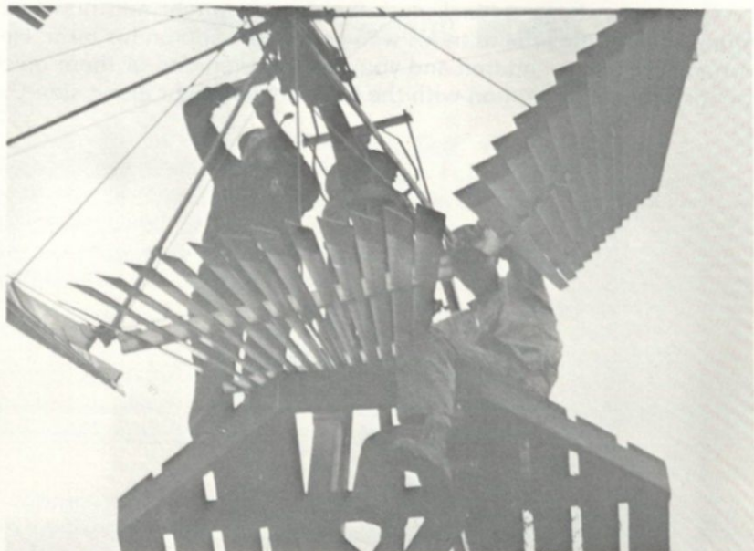
Windmill repairing by Harold Hansen and David Hanson. This is a 14 ft. wheel and is made for power instead of pumping water like most windmills.
