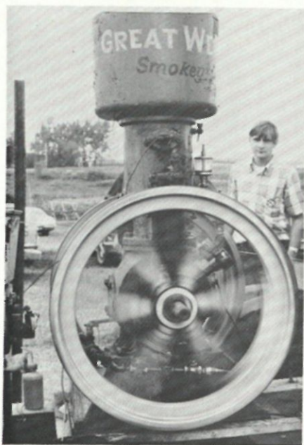
Great Western upright gas 2 cycle engine. Very few were used in our area. 4 horse power.
