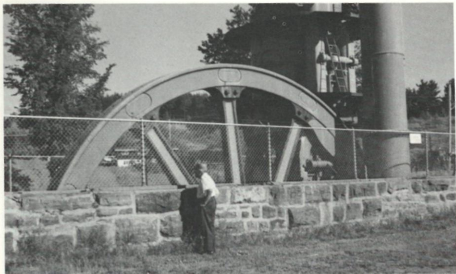
Pumping engine used in pumping water from the mines at Iron Mountain, Mi. The cylinders are high pressure 50 inches, low pressure 100 inches. Has a 120 stroke, 11 r.p.m. Pump rods were 8 inches in diameter and 7 inches in diameter. 28 inch pump cylinder, 28 inch discharge. Pumping 3400 gallons per minute or 5,000,000 per day. Flywheel is 40 ft. diameter. Weight of the engine, 160 tons.
